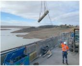
The Keepit Dam project was a \$100M+ upgrade to ensure compliance with contemporary safety standards. Part of that included installation of 52 posttensioned anchors in the spillway piers and crest. Decotec's scope included coring up to Ø350 x 11m deep and DTHH drilling 17m deep.
